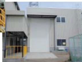
Exterior view of the liquid waste treatment building
